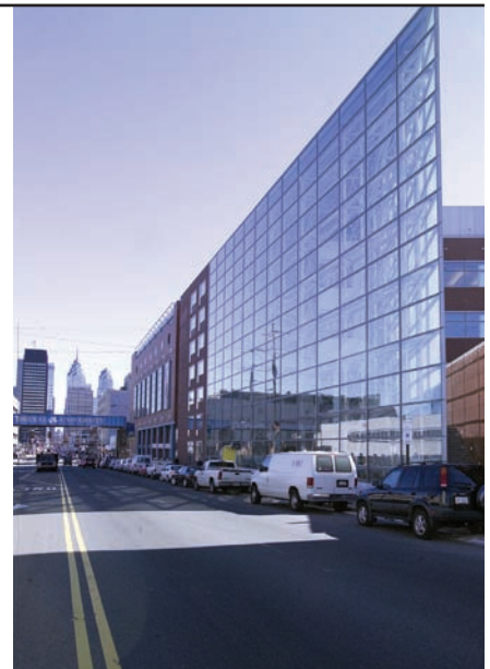
Philadelphia's Drexel University recently started using a computer system to manage a cooling system in the Bossone Research Center.
